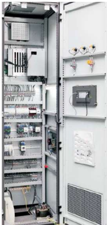
Fig 3.8 Layout in the control cabinet
